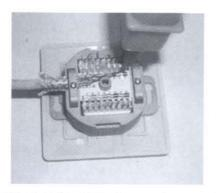
Use the 110D& KRONE impact tool to punch and connect the wires.
