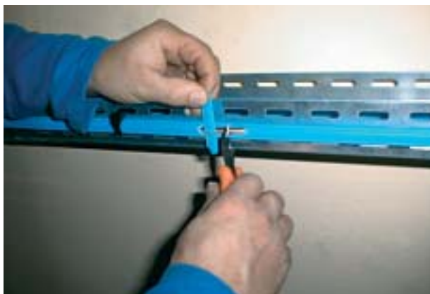
Cutting the compact tube outside the cable
