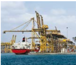
CRANES & OVERHEAD CRANES
