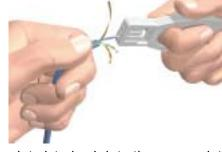
Insert each twisted pair into the appropriate slot. Rotate the tool and/or the pair in the direction opposite of the twist to prevent stripping the conductor insulation. Continue insertion to match the desire length of untwisted section.
